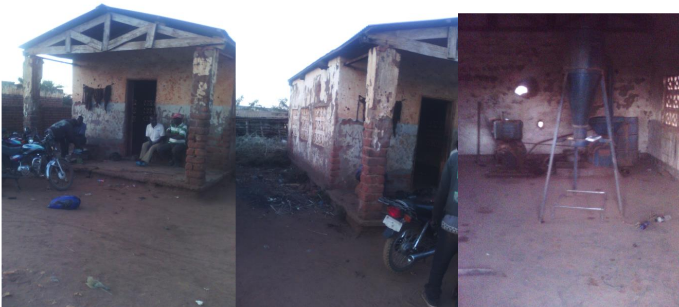
Side elevations of the abandoned building and the diesel maize mill inside
